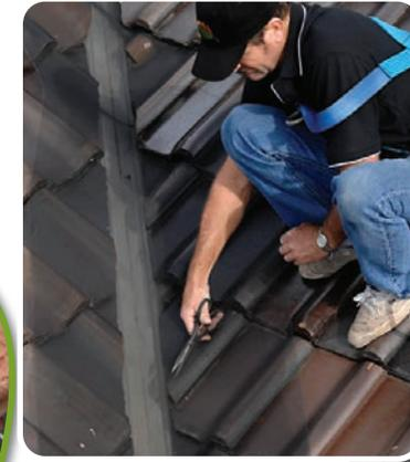
1. Cut along the ridge of the tile. The mesh will sit on the top of the tile against the ridge of the tile.
